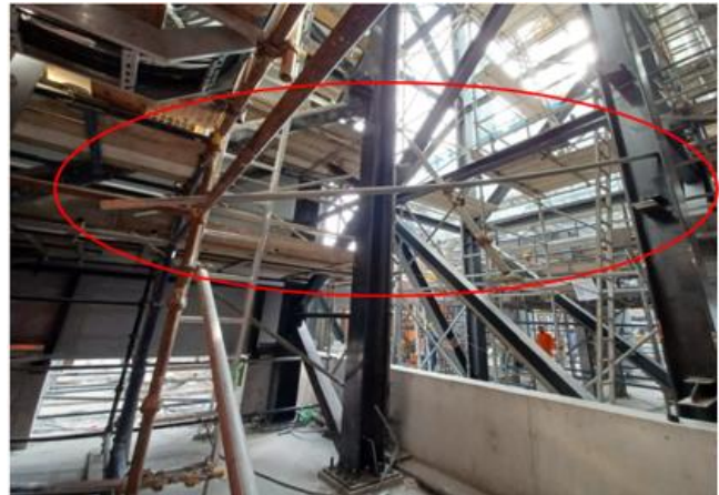
Mid rail and puncheon final landed position
